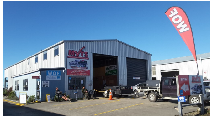
Motueka Vehicle Testing Station
